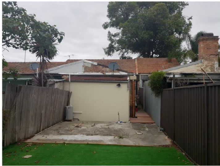
Plate 9: Rear of property showing no chimney present (note chimney on adjacent property at 89 Smith Street).
