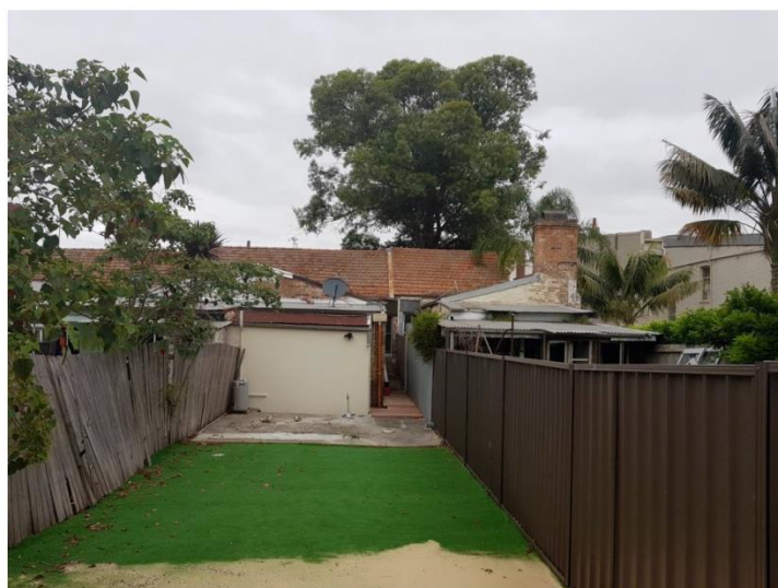
Plate 6: View of rear of house from yard.
